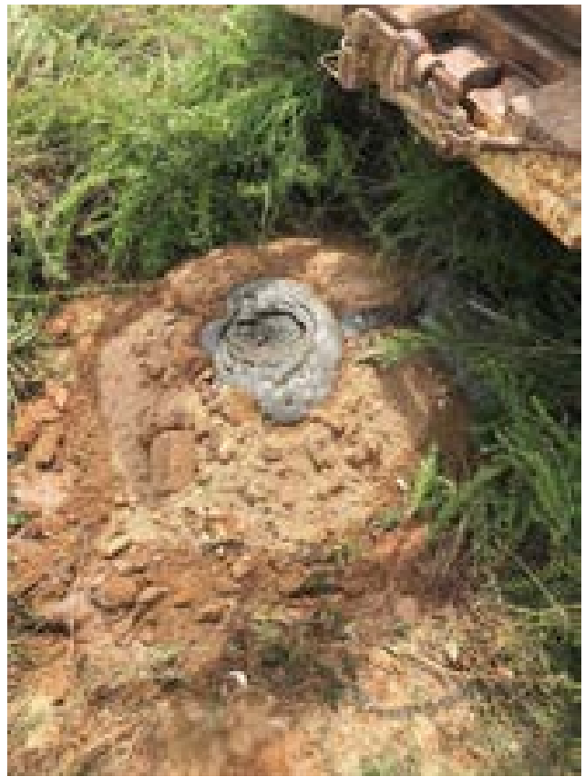
PZ-06S SURFACE COMPLETION-POST ABANDONMENT
