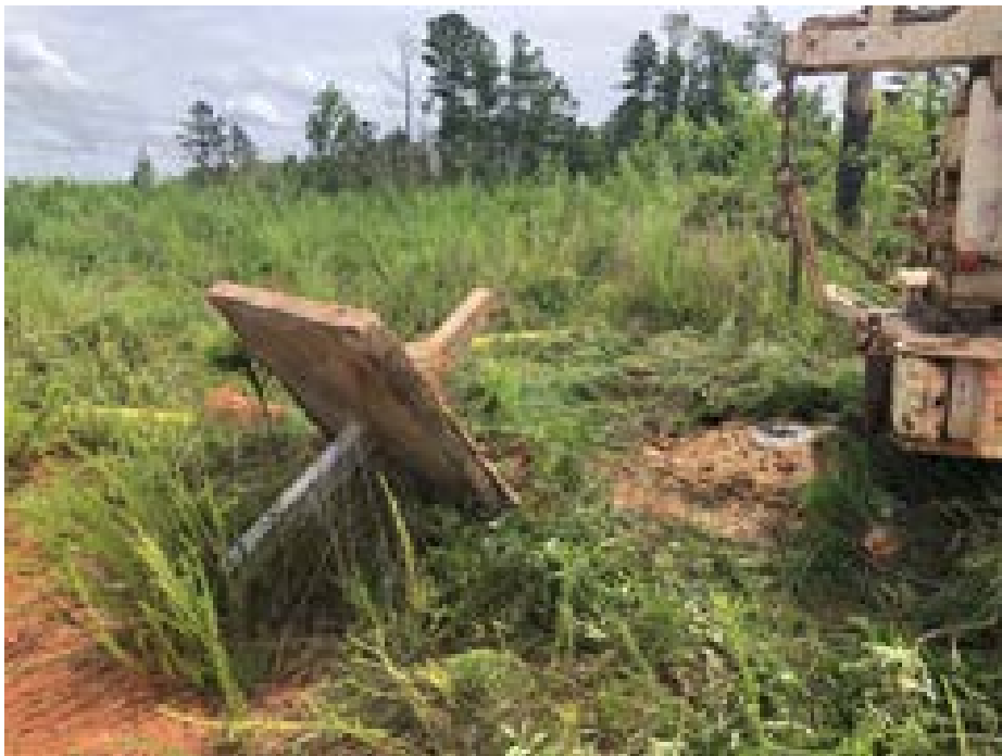
PZ-06S PROTECTIVE COVER REMOVAL /PIEZOMETER ABANDONMENT
