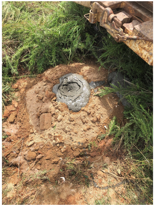
PZ-06S SURFACE COMPLETION-POST ABANDONMENT
