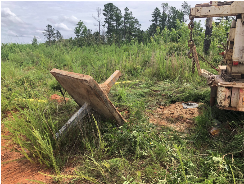
PZ-06S PROTECTIVE COVER REMOVAL /PIEZOMETER ABANDONMENT
